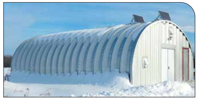
The Deep Roots Food Hub recently constructed this vegetable storage facility near Shirley's Bay
